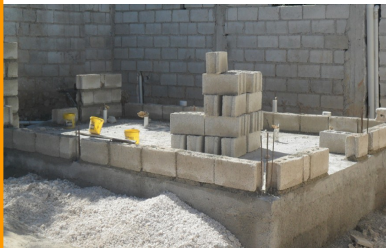
Construction of school bathroom
